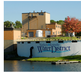
Memorial Parkway Treatment Plant
